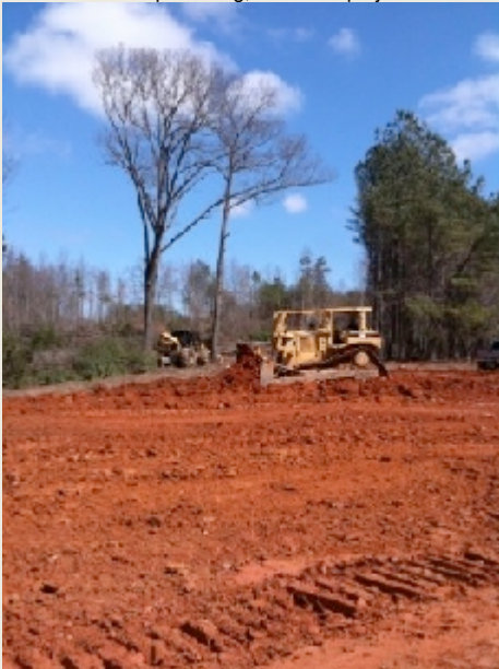
Work at the site earlier this year shortly after groundbreaking.
